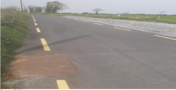
Figure 2.9: Reinstated road at joint bay (darker tarmac) with communications chamber
