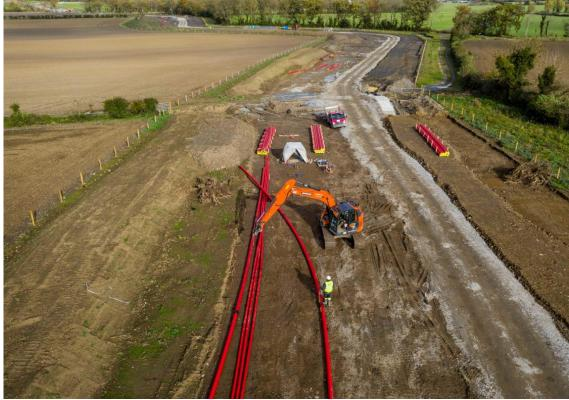
Figure 3.3: Typical underground cable construction in agricultural lands
