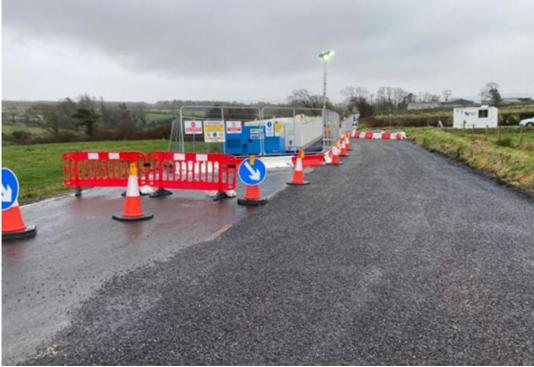
Figure 3.7: Operational Joint Bay with Passing Bay (on the Kilpaddoge Knockanure 220kV UGC Project, Co. Kerry – refer to Section 2.2.3 of the Volume 2A Planning Report)
