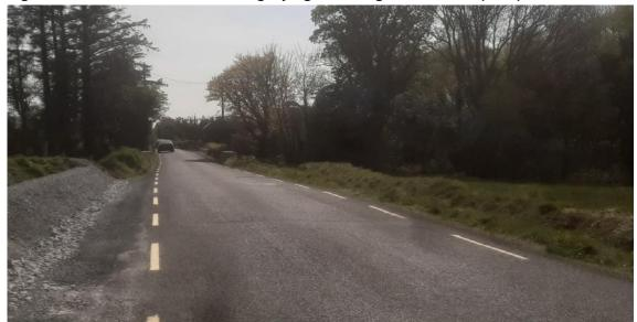
Figure 3.2: Reinstated road following laying of underground cables (UGC)
